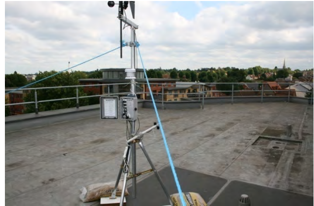
Figure 3.5: AWS Crown House
