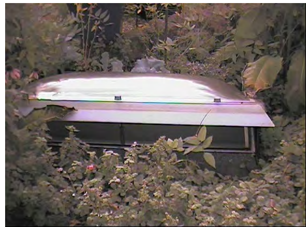
Figure 4.22: Intensive green roof - Visible image 3
