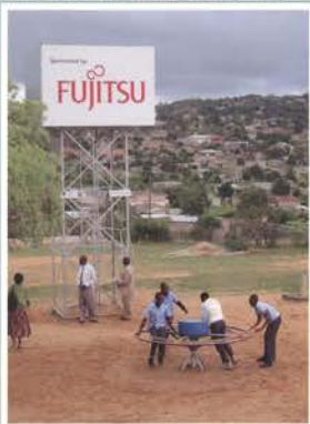
Your donation of £350 contributed to this Roundabout PlayPump. With the children play, water is pumped into the water tower and is available to them at any time. The Pump was installed at the Mankosi primary school, east of Worcester in South Africa in June 2010. 1307 children now have a fresh, clean and safe water supply for the first time!
