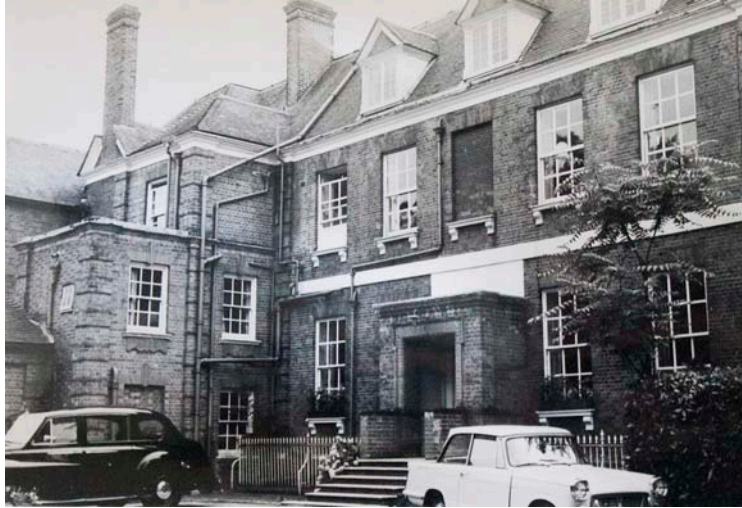
Grove House when it was part of The Grove Secondary School
